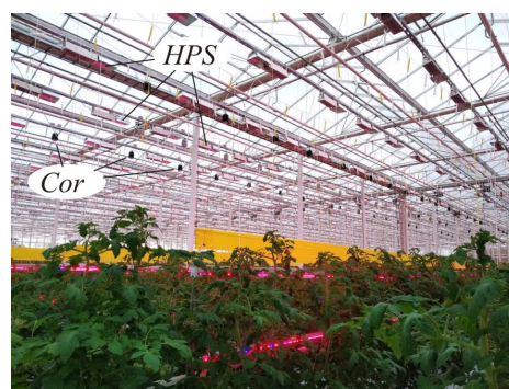
Fig. 2. Hybrid irradiation facility in the greenhouse
